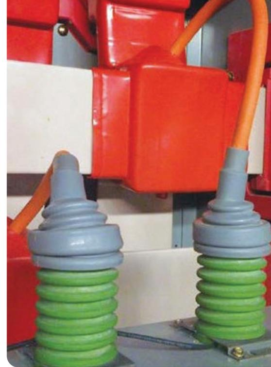
room computer or an Ethernet LAN/WAN. Switchgear and IPB not previously equipped with Iris Power capacitive couplers must have the 80 pF PD sensors installed during a suitable outage.
